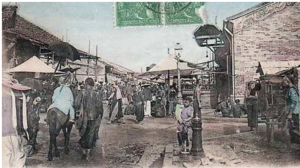
Figure 2. A Chợ Lớn Street Scene
